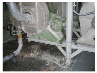
Fans installed so that vibration is not transmitted to the bearing plate
