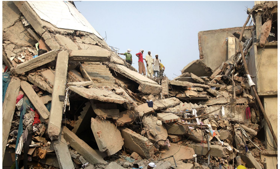
Ten years ago, the Rana Plaza textile factory collapsed, killing more than 1,100 people. The DGUV helped set up accident insurance for the textile and leather sector.
